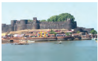
Vijaydurga Fort, Sindhudurg
