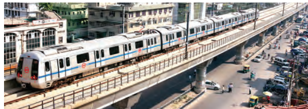
Jaipur Metro Rail
