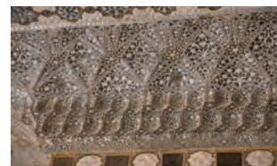
Work on Diwan-e-Khas, Red Fort
