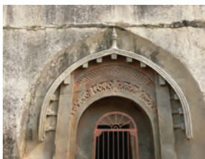
Mauryan Structure at Barabar Caves
